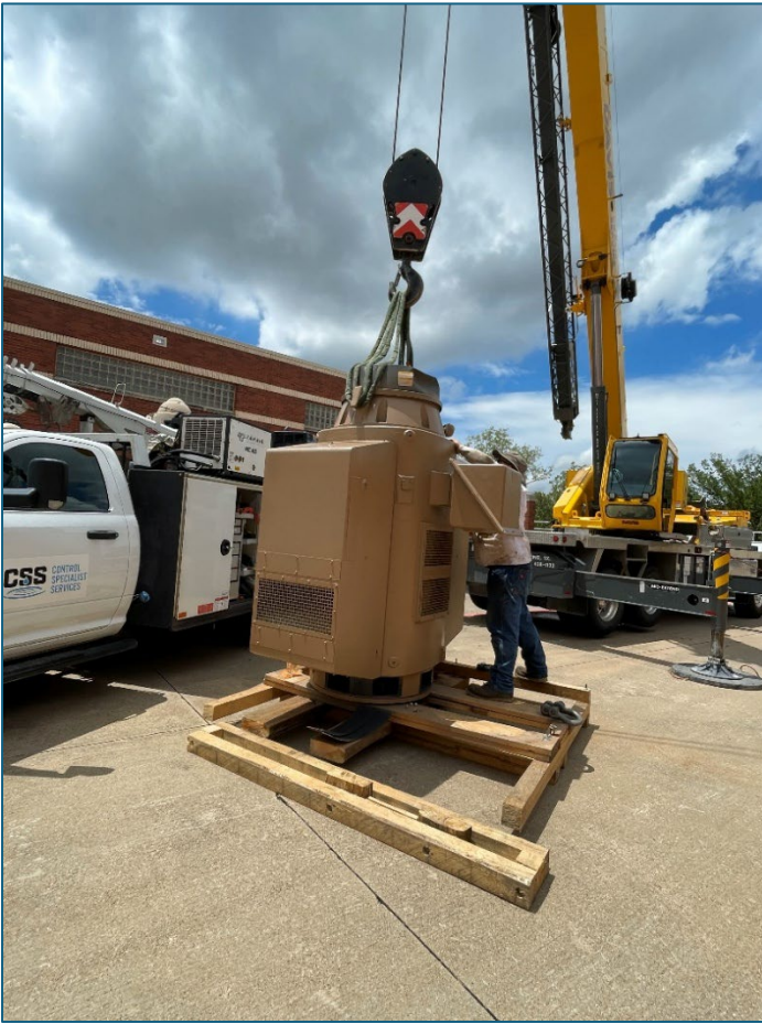
Lowering the motor into place.
