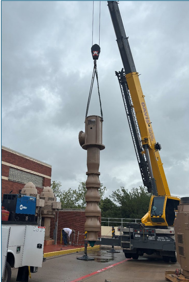
Lowering the pump into place.
