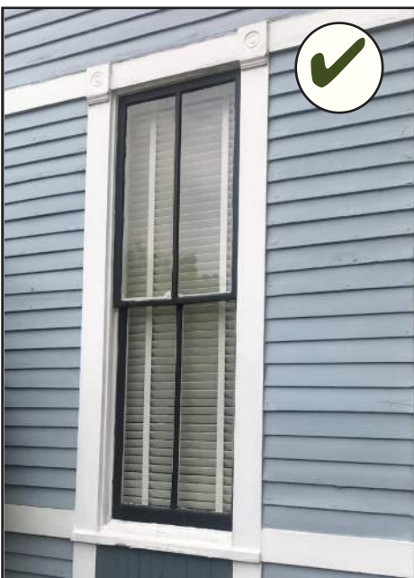
This two-over-two wood window, with an appropriate trim, is an excellent example of a well maintained window in the district.
