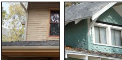
Weatherboard siding
