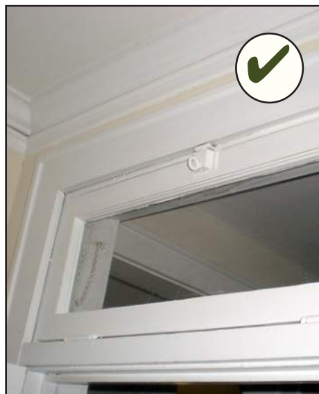
Transoms allow passage of air and light between rooms even when doors were shut.
