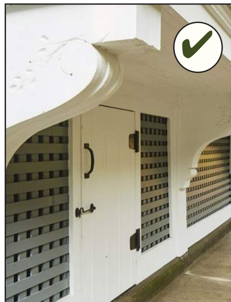
Square wood lattice panels are the preferred pattern for this type of wood skirting in the district.
