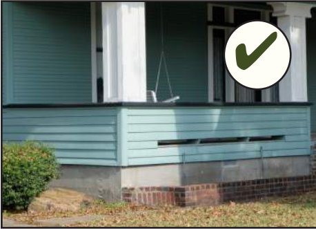
Protect exposed foundations with appropriate materials such as wood skirting or lattice, concrete, brick or metal flashing, or pressed metal.
