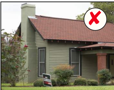
Paint or stucco is inappropriate for masonry chimneys that were historically unpainted or not stuccoed.
