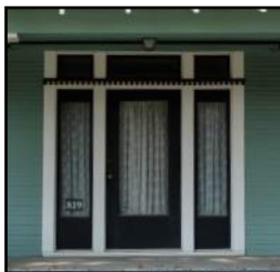
Partially-glazed, single door with side lights and transom.
