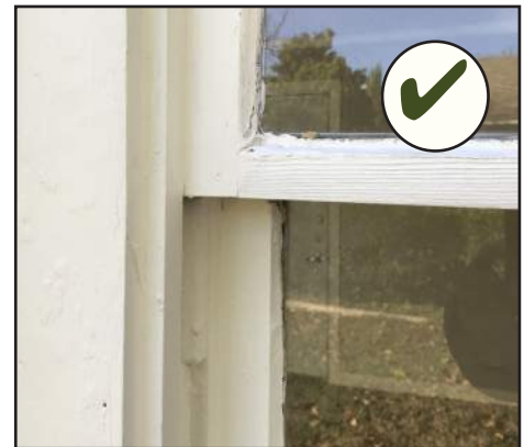
Detail of wood window sash on a window maintained in its original condition.
