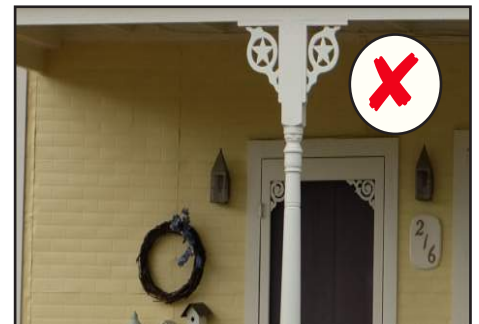
This siding on this historic building has been replaced with yellow-painted, pressed-metal siding made to look like brick. This is not compatible with the historic building and can cause damage to the historic fabric.
