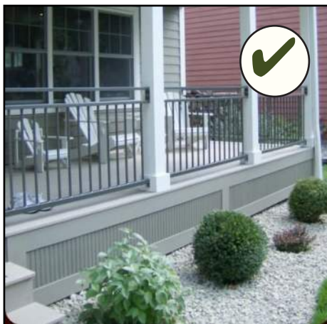
This foundation height and skirting material are compatible with the architectural style of the house and would be compatible for the district.
