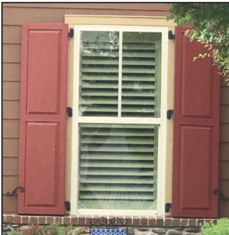
Operable shutter installed at the window jamb.
