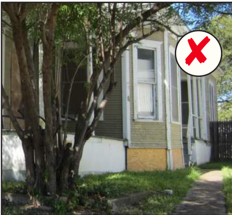
This plywood foundation skirt is an inappropriate material for Haggard Park and would not have historically been found on buildings in the district.
