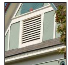
Louvered window for ventilation.
