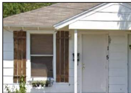
Existing masonite siding on a minimal traditional style building in the district.
