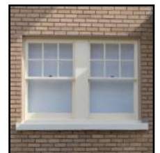
A pair of six-over-one, double-hung windows. Both sashes are operable.
