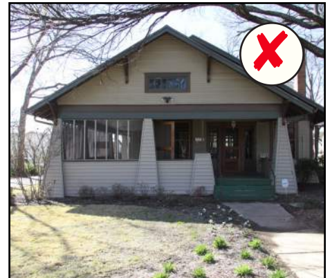
The porch columns and siding have been wrapped in metal, an inappropriate material for a Craftsman-style house.
