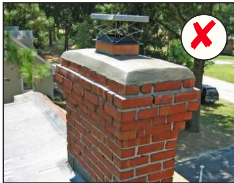
Dampers should not be installed on chimneys.
