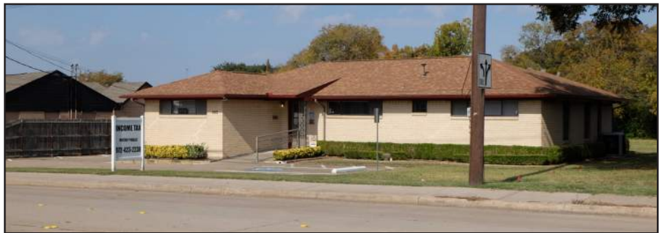
Roof form, like the low-pitched, hipped roof on this Ranch-style building, are character-defining features.
