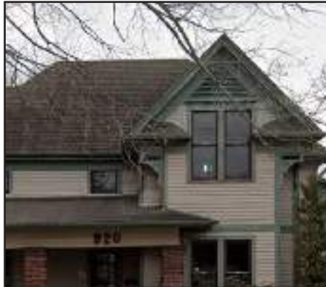
Roof features, including pitch and gables, are character-defining and should be retained.
