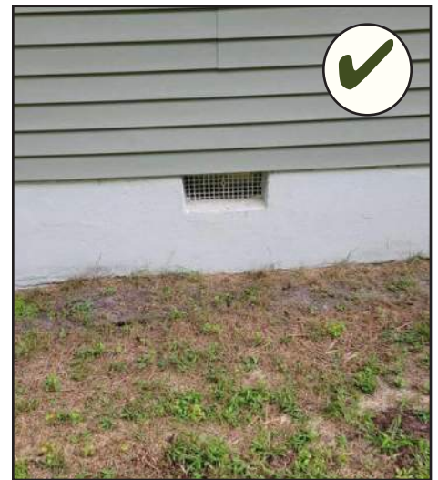
Crawlspaces in historic foundations should have vents for adequate ventilation.
