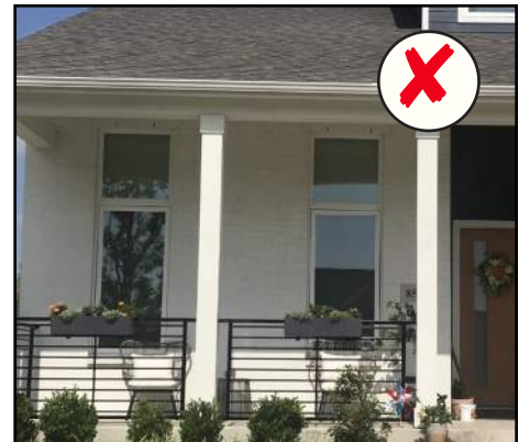
These one-over-one windows are not proportional between the window and the transom above and are therefore inappropriate for Haggard Park.
