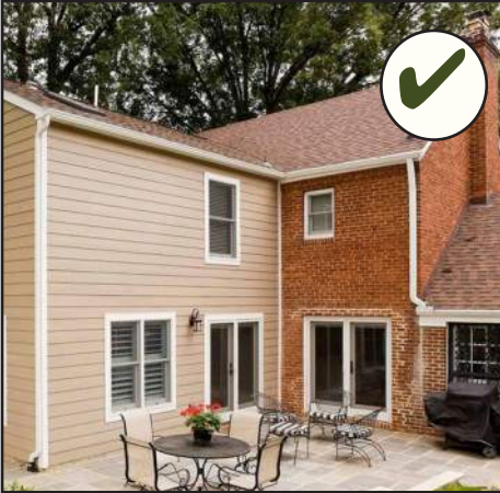
This addition has differentiated materials of wood siding and brick which are compatible.
