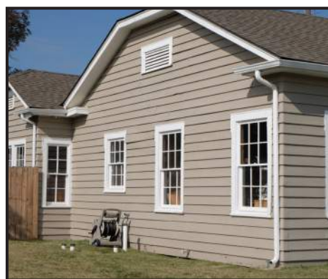
Avoid stripping exterior paints as it can cause damage to the wood siding.
