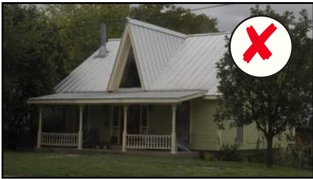
The steep pitch of this front dormer addition is inappropriate for the style of this house. Most of the roofs in the heritage district have low- to medium-pitched roofs.
