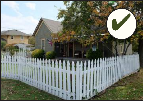
If a front yard fence is desired, construct historically appropriate, compatible fences. Wood fences shall be at least 50% open and not exceed 40 inches in height.
