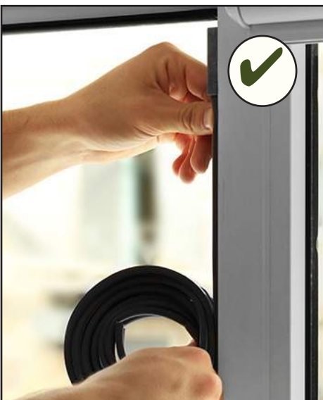
Weatherstripping can help seal air leaks in areas of your home, such as doors, windows and attic access points.
