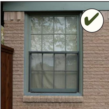
Maintain and repair historic windows to retain energy efficiency. Weather-stripping may be added to improve efficiency.
