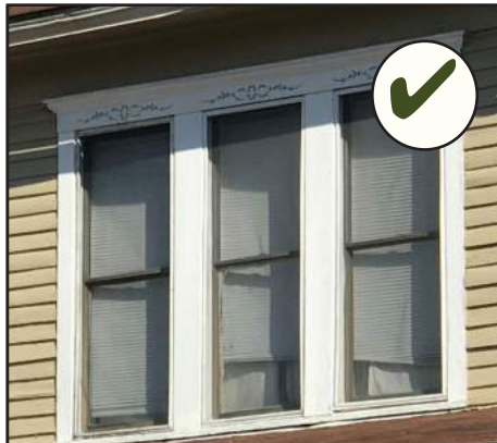
Detail of a wood window, showing appropriately maintained trim, screens, and proportion.
