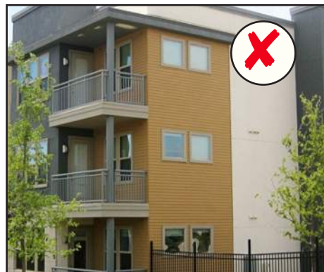
Townhouses and multi-family units, if allowed by Zoning, must have a residential form with sloping roof. This flat, projecting roof, as well as other features of the building including cantilevered concrete balcony and metal siding, are inappropriate for the district.
