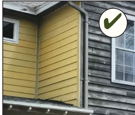
Smooth finish cementitious board, shown here next to existing wood siding, is compatible.
