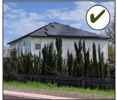
Install solar panels on the same plane as the roof with compatible colors.
