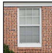
A six-over-six, single-hung window on a Ranch-style house. Only the bottom sash is operable.
