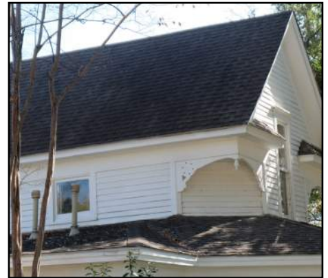
Existing roofing materials in Haggard Park are typically composition shingle.
