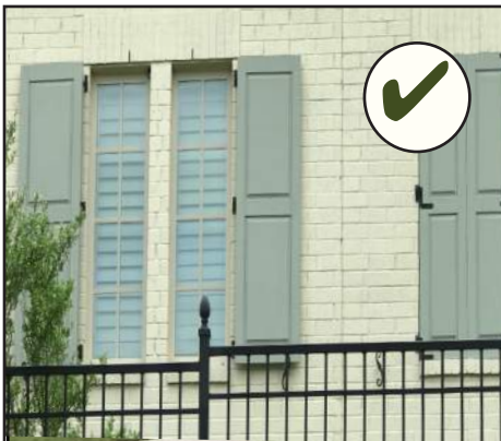
Windows with attached shutters that are operable are appropriate for the heritage district.
