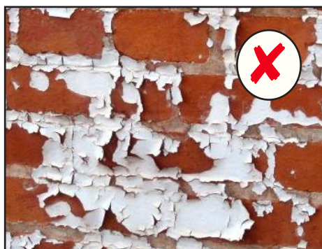
Non-historic paint coatings and water repellent treatments are inappropriate for historic masonry.
