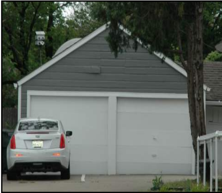
Wood siding on accessory buildings in the district may be painted, opaque stained, whitewashed or "weathered wood".
