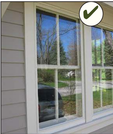
Storm windows can help reduce air movement into and out of existing windows, reducing heating and
