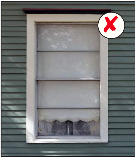
Windows shall not be replaced with incompatible materials, such as the replacement of wood windows with aluminum, as seen here.
