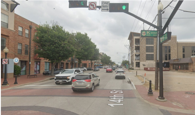
Facing east from K Avenue towards Municipal Avenue
