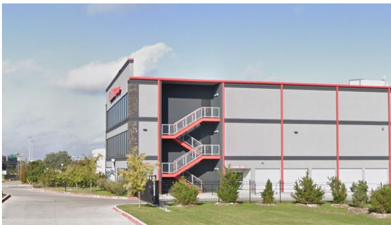
Left: Mini storage building with a parapet wall.
