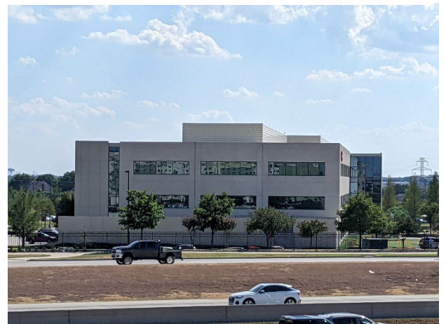
Right: Office building with rooftop screening.
