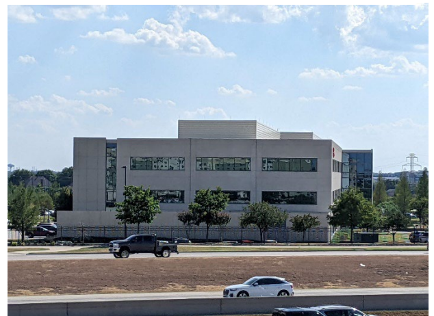
Right: Office building with rooftop screening.
