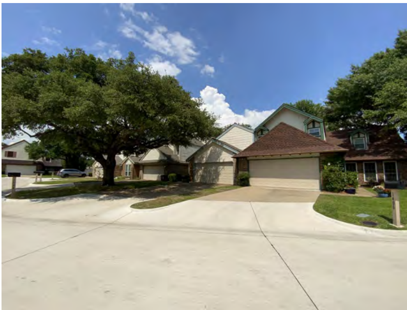
Figure 64. Photograph of the townhouses in Wood Park #1.
