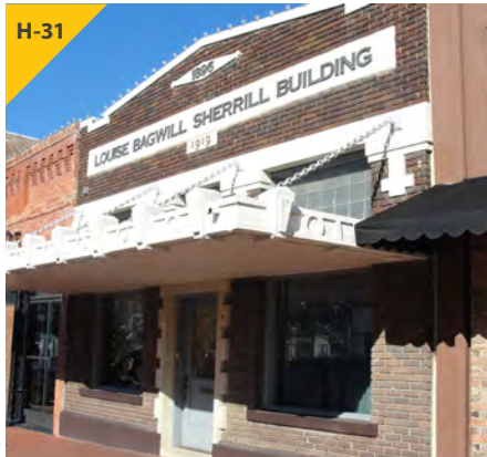
H-31 Bagwill-Sherrill Building 1015 E. 15th Street Constructed: ca. 1895/1919 Style: Art Deco
