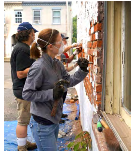
Restoring a historic brick building
