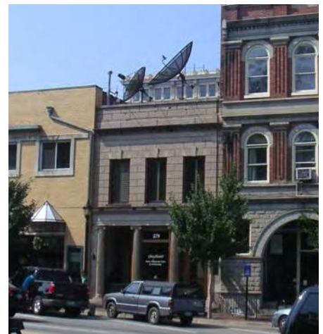
Satellites added to the roof of a historic building
