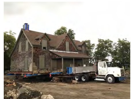
The Fox-Haggard (Collinwood) House was moved from its original site to a new location prior to construction of Windhaven Meadows Park.
