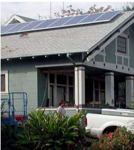
Solar panels on a historic building
