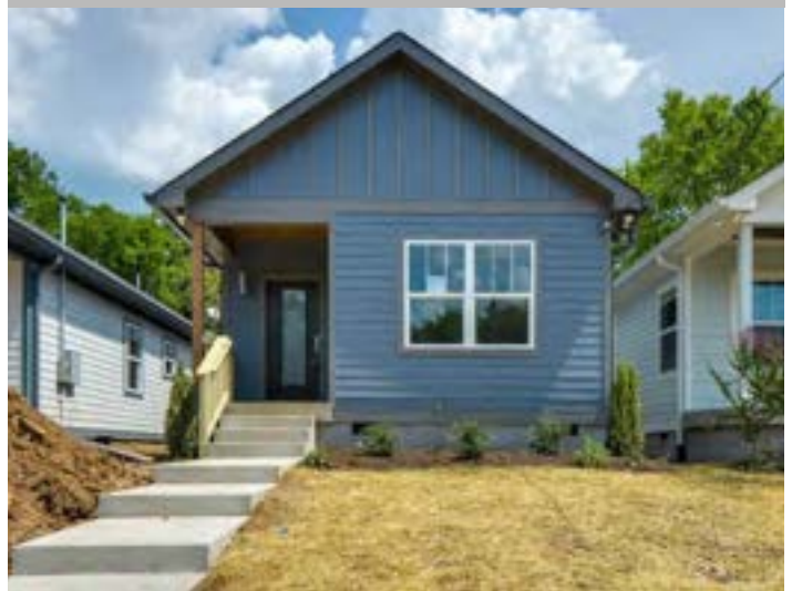
Existing Douglass Community detached single-family housing
