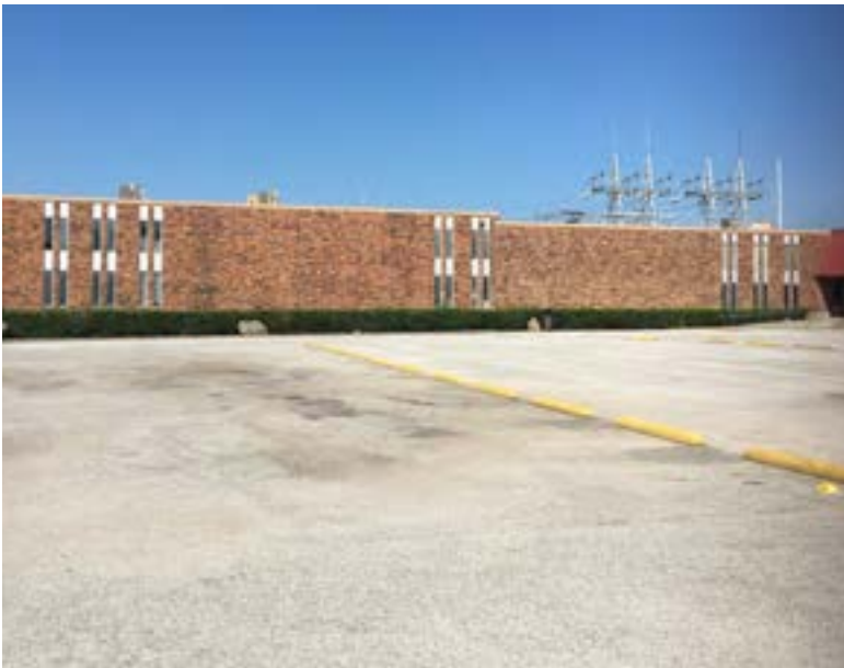
Light industrial uses
