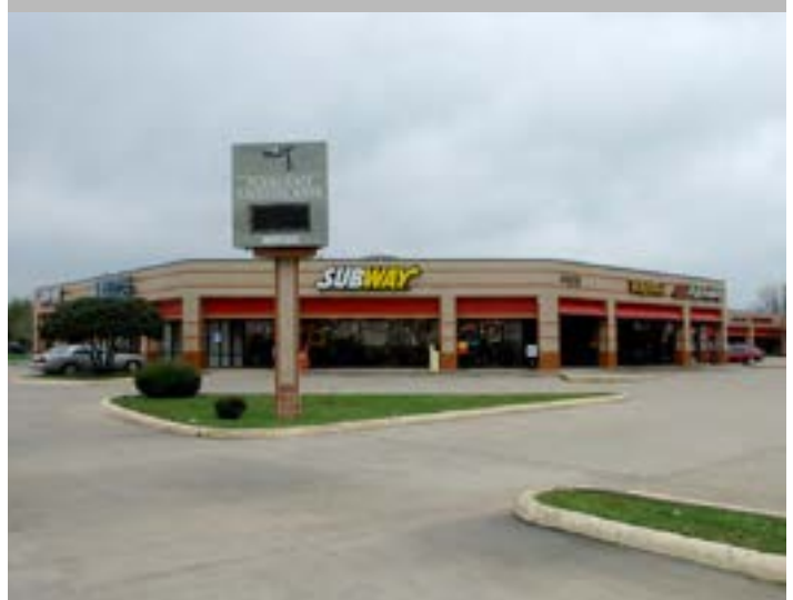
14th Street corridor retail development
