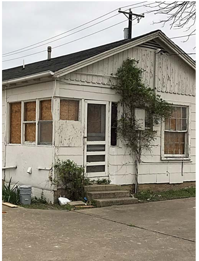
WEST ENTRY DOOR
