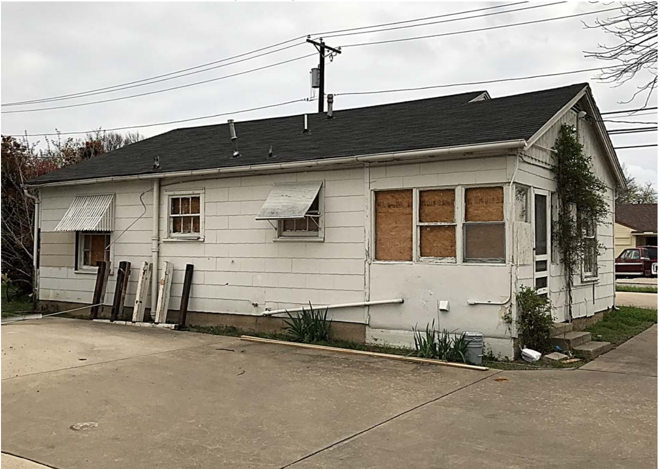
REAR (NORTH) FACADE
