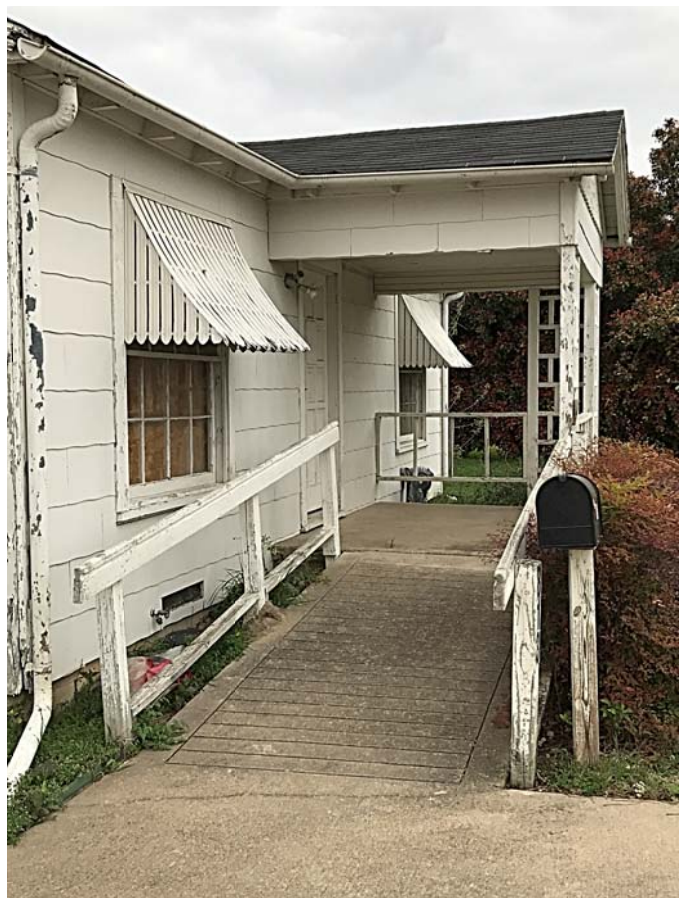
ACCESSIBLE RAMP AT FRONT
