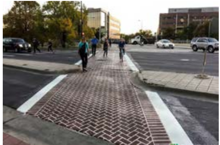
Decorative intersection treatment
