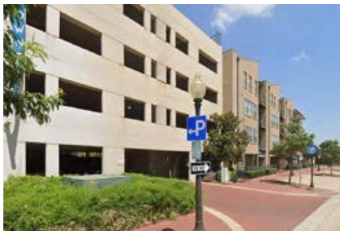
Downtown Plano public parking garage
